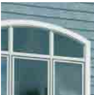
Restoration Millwork trimboards can be heat-formed to create arches around windows.
